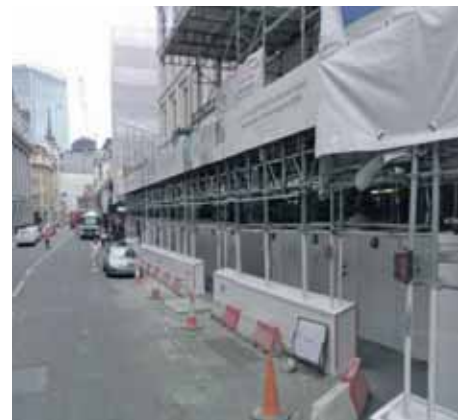
Under construction, the rank remained in place throughout the building works.
